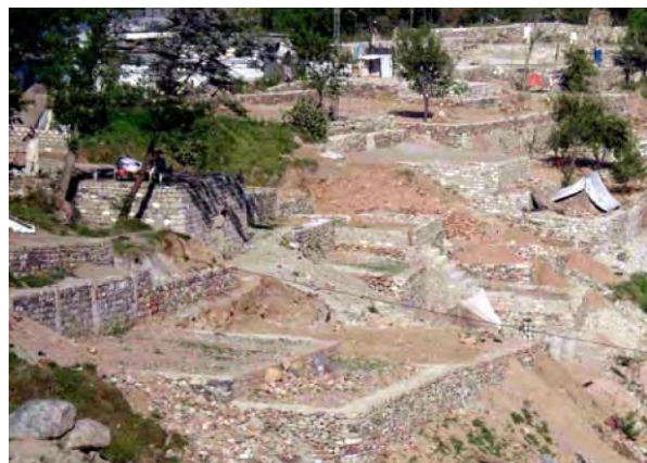
Constructed retaining wall
