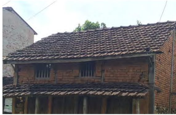
Clay tile roof
