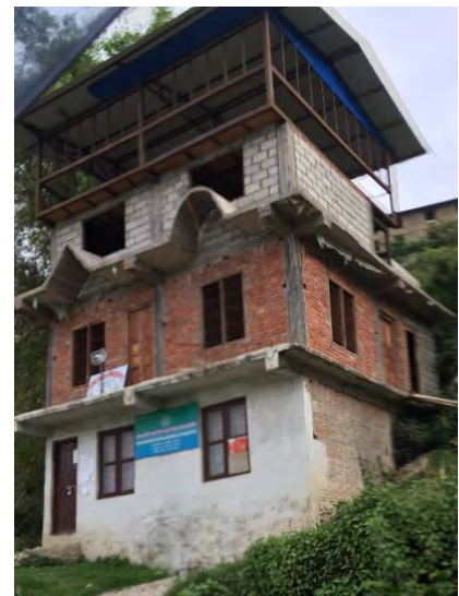
Mix-use of stone and brick for masonry wall
