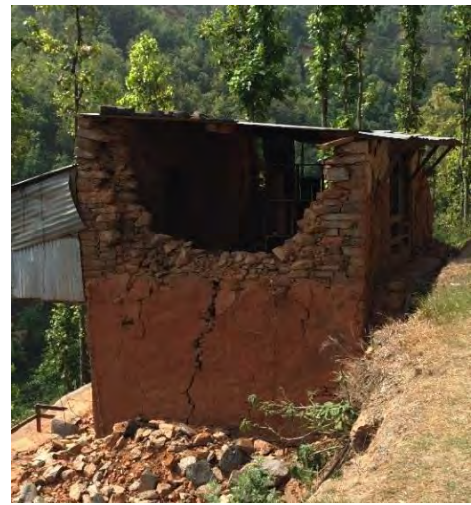
Damage of stone masonry gable wall
