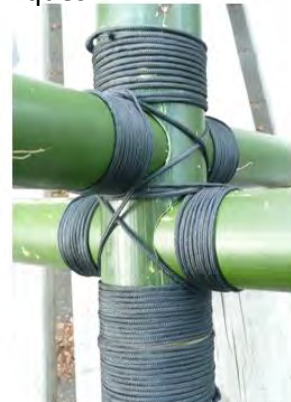
One Vertical, Two Horizontal members fitting connection combined with lashing technique
