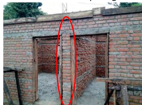
Distance of opening from the wall corner
