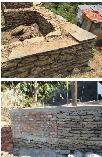
Mix-use of stone and brick for masonry wall
