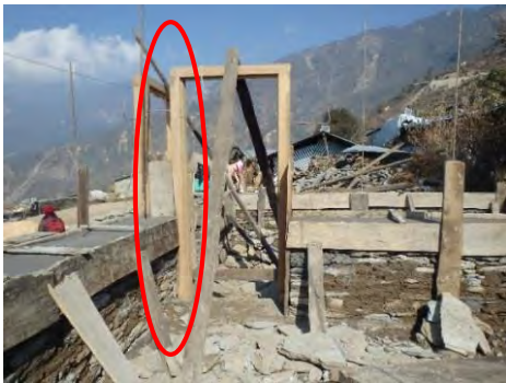
Opening attached to the edge
