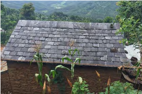
Slate stone roof
