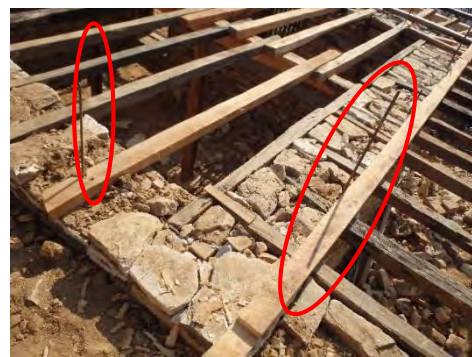
Vertical reinforcement provided at different location
