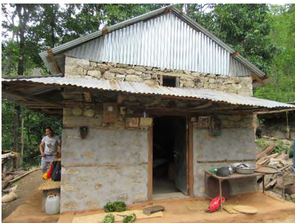
One+Attic by stone masonry in mud mortar with wooden band
