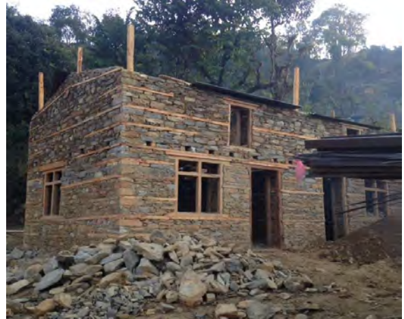
Two storeys constructed by stone masonry in mud mortar.
