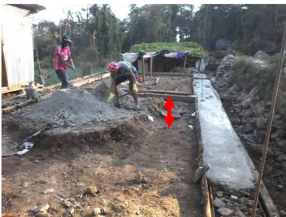
Level of plinth is less than 300mm from ground level
