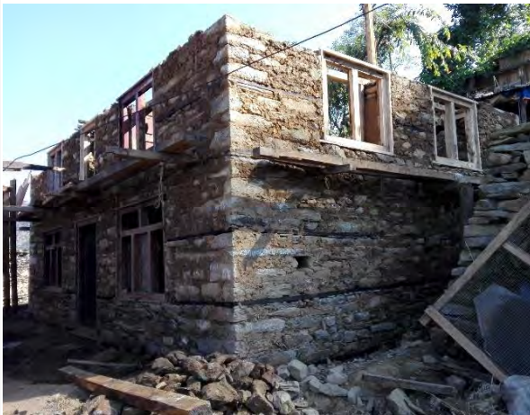
Two storeys constructed by stone masonry in mud mortar.
