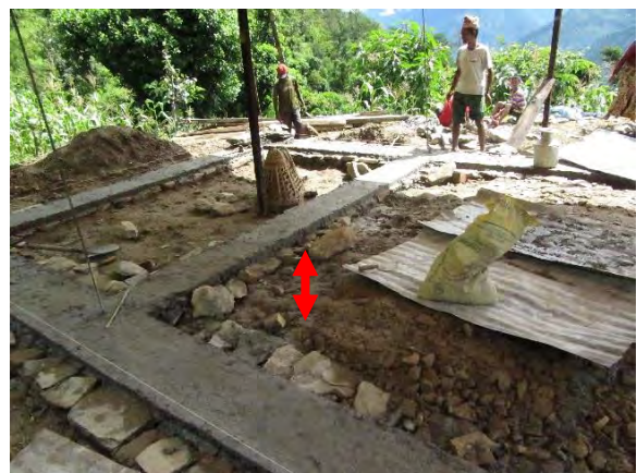
Level of plinth is less than 300mm from ground level
