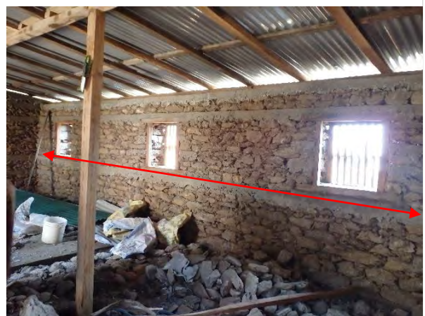
Span of wall is more than 4.5m
