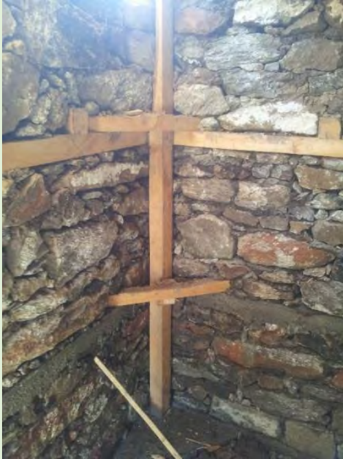
Details of wooden diagonal bracing
