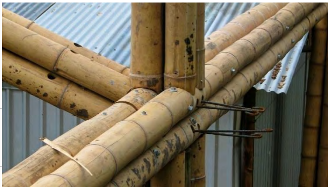
Vertical, Horizontal & Diagonal members connection using GI Wire (10 Gauge)
