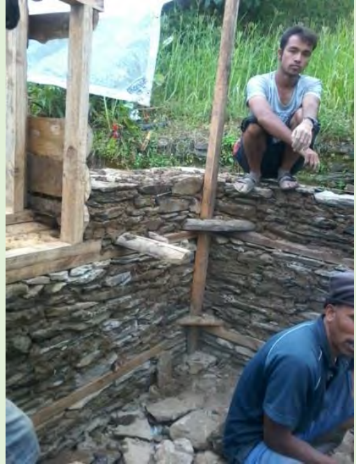
Details of wooden diagonal bracing
