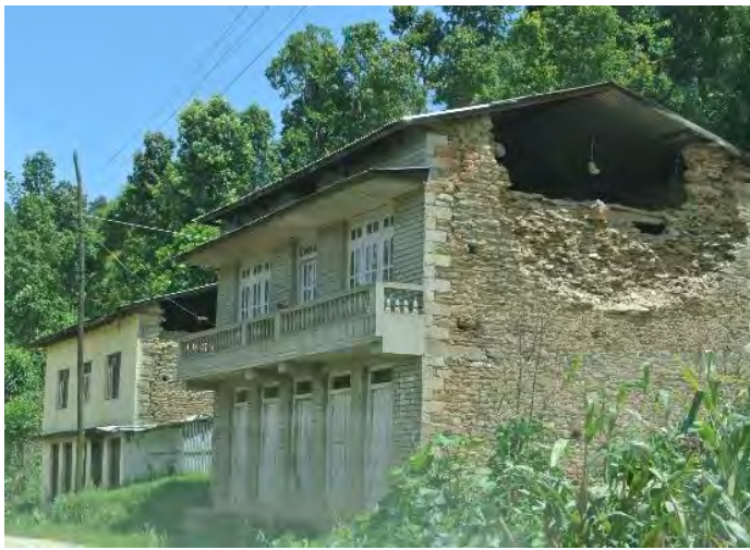
Damage of stone masonry gable wall
