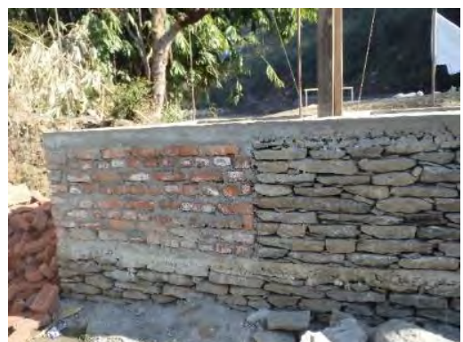
Mix of materials used in masonry walls
