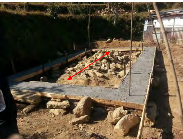
Span of wall is more than 4.5m
