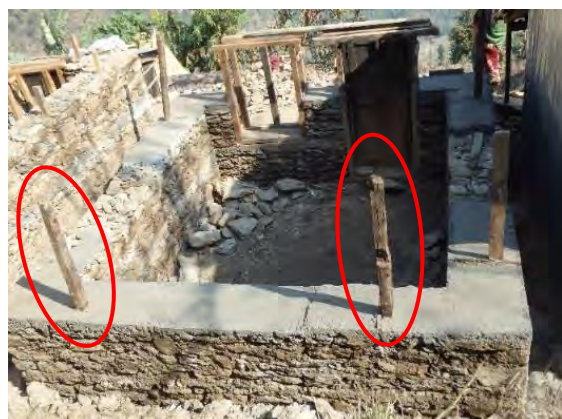
Vertical band provided in different locations
