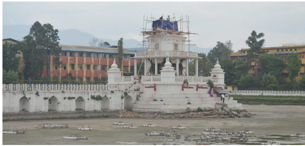
Reconstruction underway at Rani Pokhari, Kathmandu.
