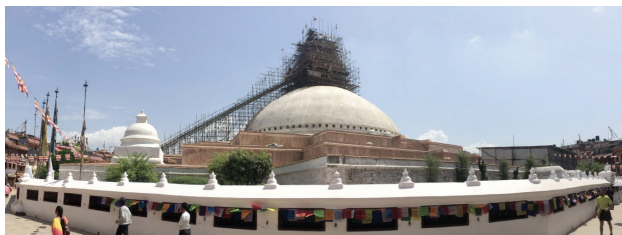
Community reconstruction of the Boudhanath stupa.
