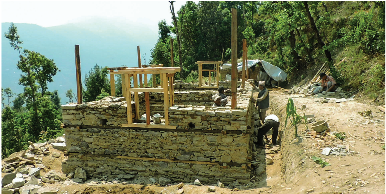
A family building an earthquake safe house in Laduk VDC Dolakha.
